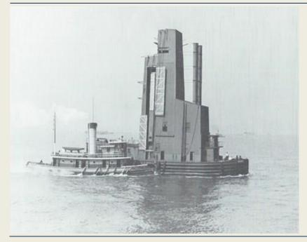
The Walter L. Meseck side towing the *Hudson*, a floating grain elevator. The Hudson was brought alongside an anchored ship and used to suck grain out of the ship's hold and discharge it into waiting barges. Undoubtedly, the Meseck would have handled the barges as well. Unlike the Hudson, many floating grain elevators were self-propelled and had limited need for tug assistance. (Source: On the Hawser by Steven Lang and Peter H. Spectre)
